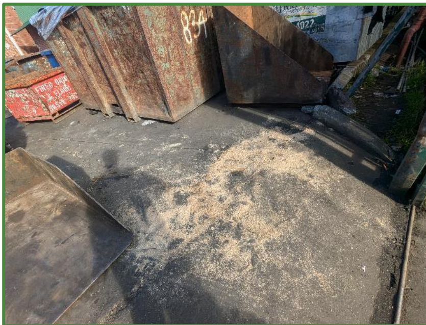
Photograph 5: Hardstand along entrance driveway. Sand/sawdust used to contain/prevent mobility of spillage visible. Various stored skip bins visible in background (viewer facing northwest).
